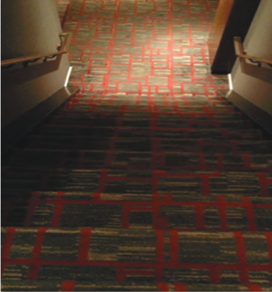
Figure: A typical carpet pattern on stairs that makes it difficult to see where one step ends and another begins. Stairs should be clearly demarcated with contrasting strips and well lit.
